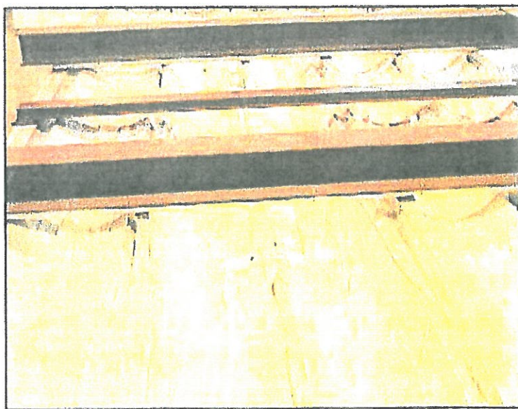
PARTIAL SEAM DISENGAGEMENT AND CLIP SCREW PULLOUT
