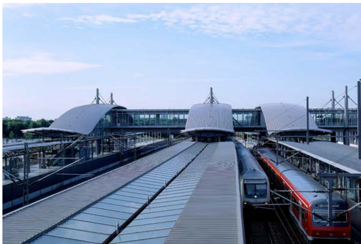
FERNBAHNHOF DÜSSELDORF, DEUTSCHLAND LONG-DISTANCE RAILWAY STATION DÜSSELDORF, GERMANY
